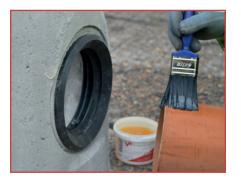
2. Chamfer the edge of the connecting pipe and lubricate.
