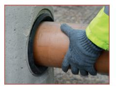
3. Centre the end of the pipe and push it into the seal, ensuring that the pipe end is flush with the inner wall.
