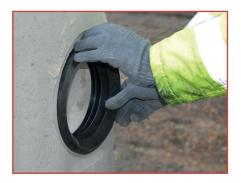
1. Insert the wall seal into the hole. Lubricant is not required.
